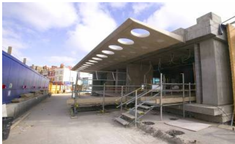
DLR Station Entrance under construction in Woolwich New Road Woolwich SE18
